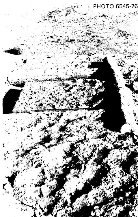
Fig. 4.6. Blast-protector logs around blast door after these logs were moved by blast effects at the 53-psi overpressure range.
